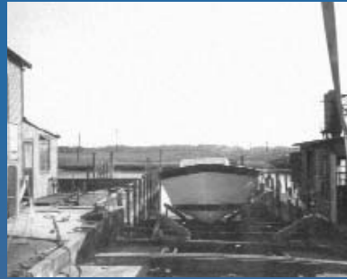
CIRCA 1965. An early Silverton Yacht fiberglass hull undergoes water-testing.
